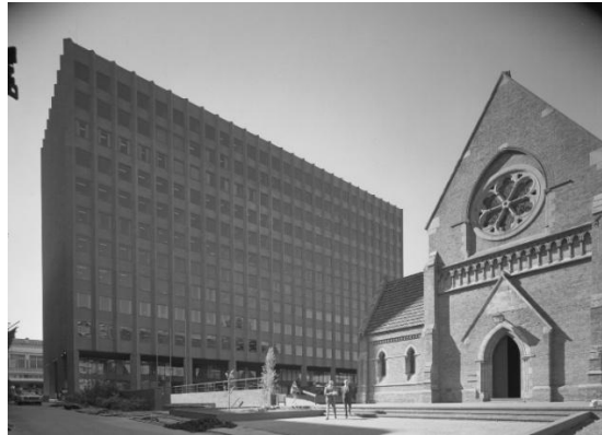
1972 Law Chambers Building centre, with St George's Cathedral at right (Fritz Kos, SLWA 160126PD)
