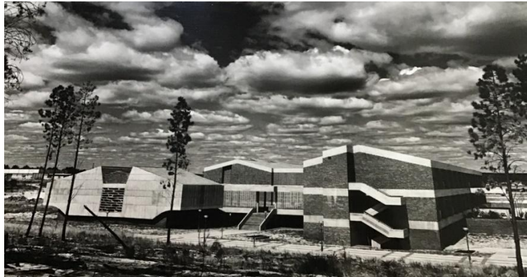
Curtin University buildings 307 at left, 306 behind, and 305 at right, circa late 1960s. Photo taken from the west, on the current location of the library (B105) opened in 1971 (Moira Russo).
